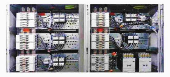
During previous decades manufacturers of automatic compensation banks faced increasing competition worldwide. They were forced to produce as economically as possible. Now, new technologies have been developed compared with the past when capacitors were bigger and heavier. Minimizing capacitors enabled the development of steps (modules containing capacitors) with discharging resistances, fuses, contactors and reactors (if required) assembled in standardized industrial cubicles.
